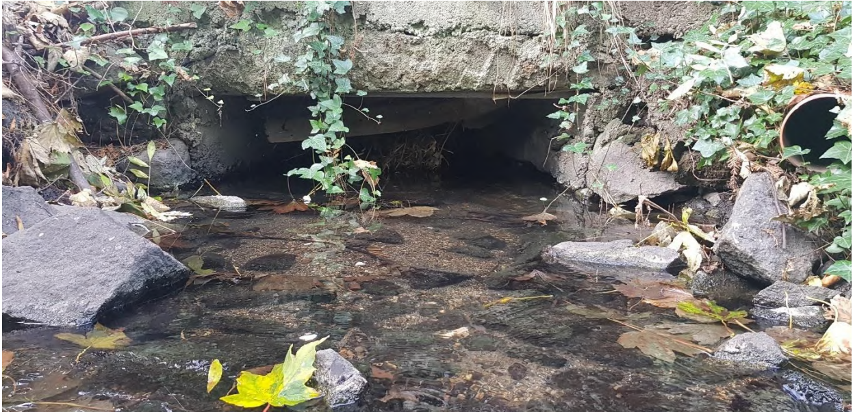
Figure 4.6: Richmond Green Culvert – Upstream Face
