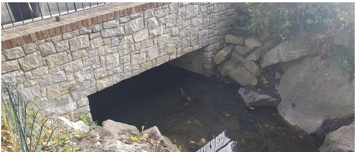
Figure 4.8: Alma Place Culvert
