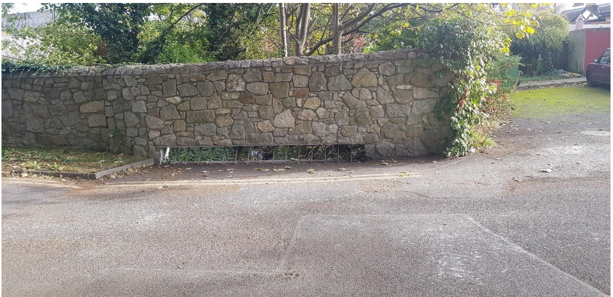
Figure 4.7: Richmond Green Culvert – Grille
