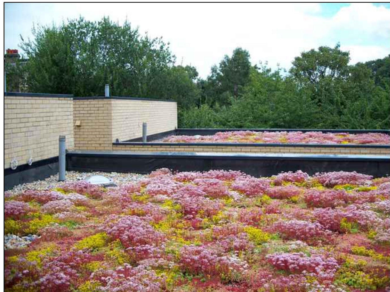
BLUE/GREEN ROOF ZINCO FIXODRAIN LAYER PRIOR & COMPLETED SEDUM GRASS APPLICATION (SOURCE: BETON CONSTRUCTION SERVICES LTD.)
