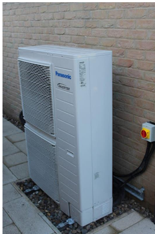
Fig. 4.4 – Typical Air Source Heat Pump Installation
